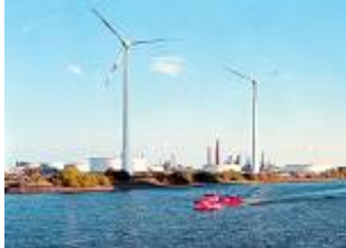
Harburg, Germany 3.6MW
