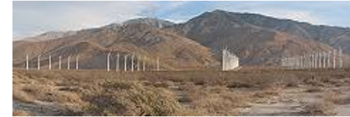
Cabazon Pass, California 41MW
