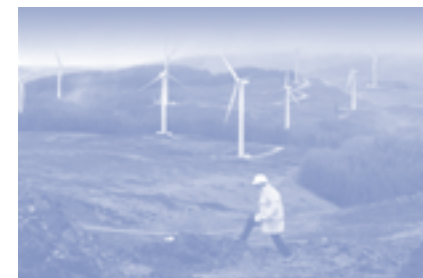
Cruach Mhor wind farm © ScottishPower
