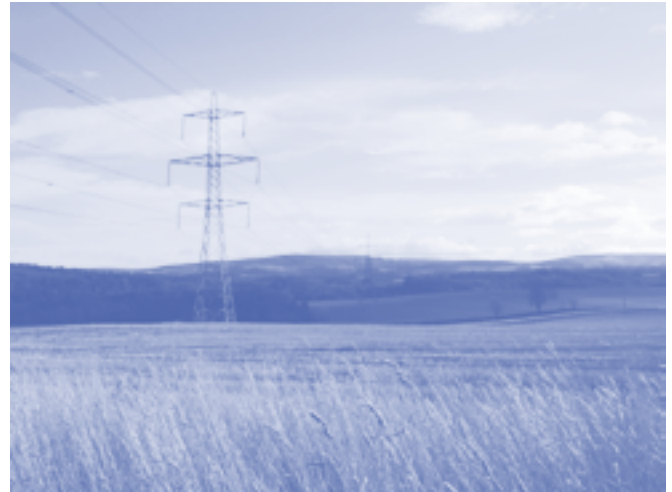
© Scottish and Southern Energy
