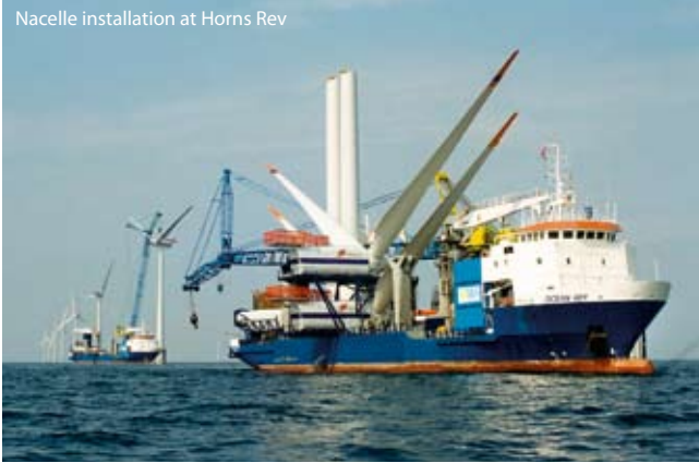
Nacelle installation at Horns Rev
