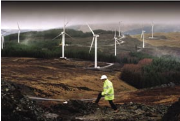
Cruach Mhor Wind Farm © ScottishPower
