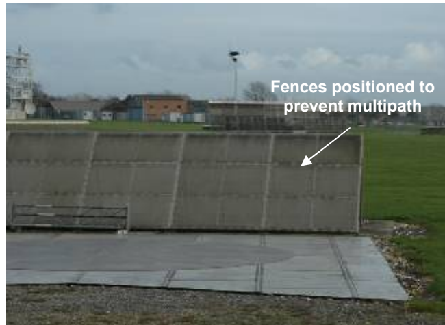
Figure 3 Fences used to reduce interference from reflections
