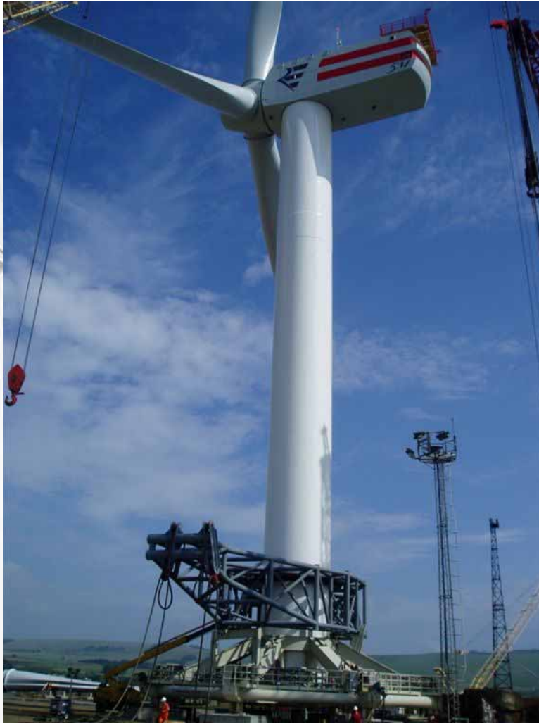
➤ The Spreader Beam in Place
