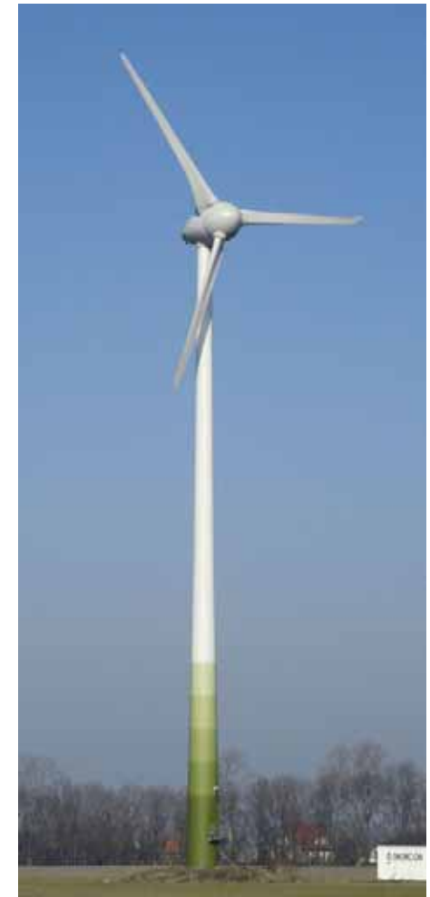
333 kW Enercon; Ø33 m, 50 m tower
