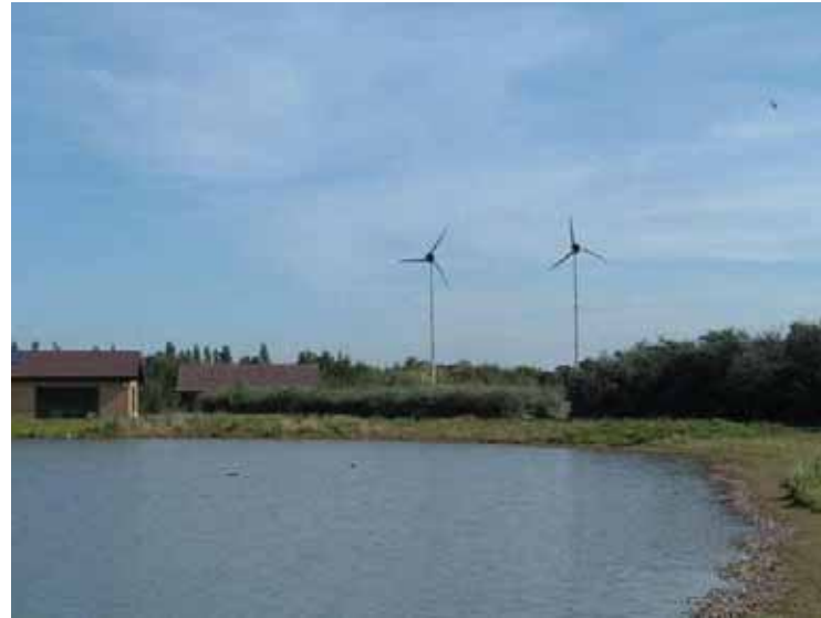
A pair of 5 kW Iskra AT5-1s; Ø5 m with 15 m tower
